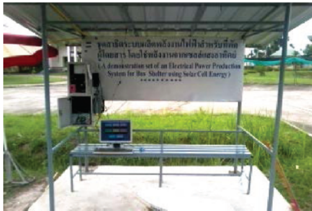
Fig. 2 The bus shelter.
