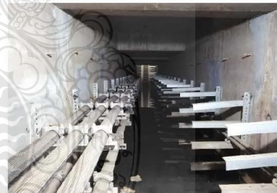
Fig.6. Square tunnel for the underground power cable installation
