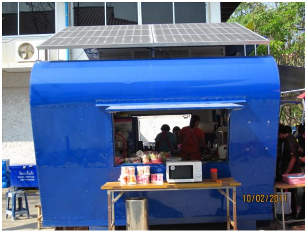
Figure 5. Installation of photovoltaic system at the roof of small food kiosk
