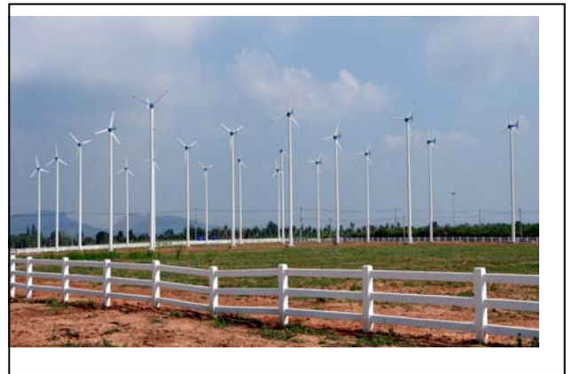
Fig.4 100 kW mini-wind farm for grid connect
