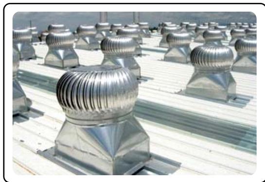
Fig.1. Roof Ventilator on the Building
