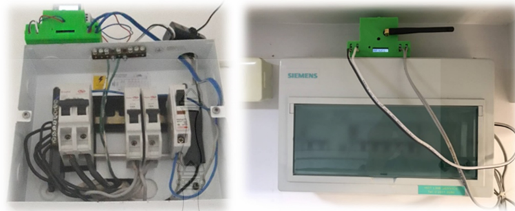
Figure 9. Installation of the NILM embedded box.
