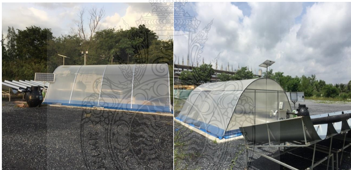
Figure 3-19: Photographs of assembling the drying system
