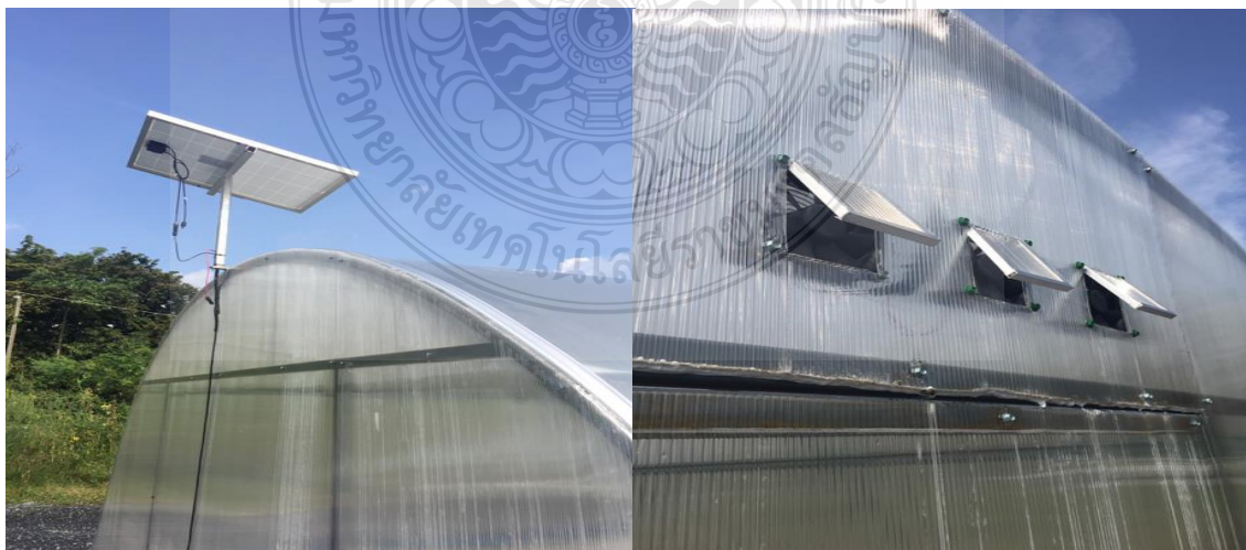
Figure 3- 9: Photographs of Installation solar panel and fans of the dryer
