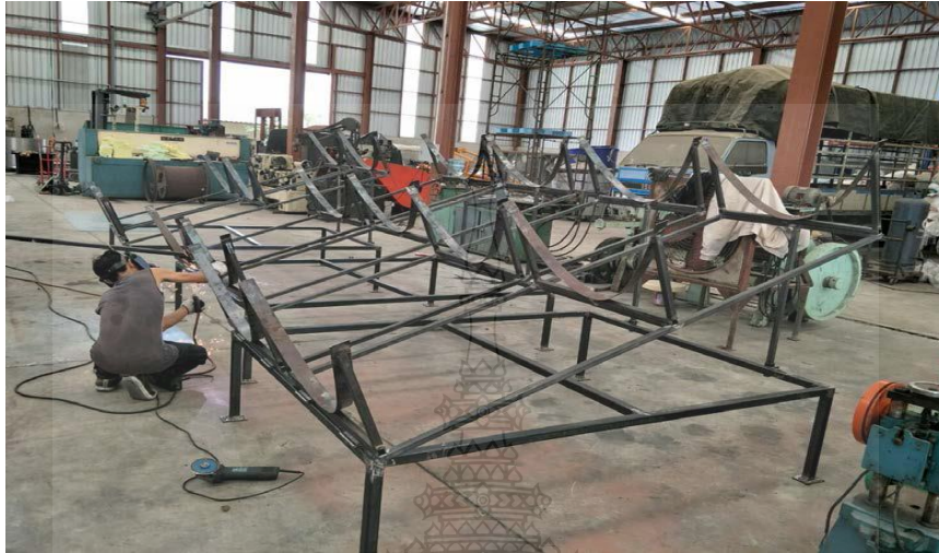
Figure 3- 13: Photograph of fabrication structure of the parabolic collector
