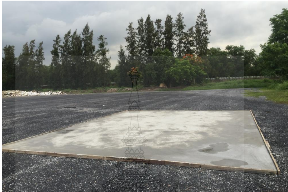
Figure 3-6: Photograph of paving concrete floor of the dryer
