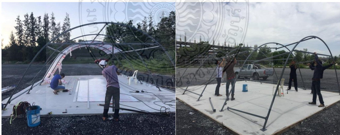
Figure 3-7: Photographs of installation structure of the dryer
