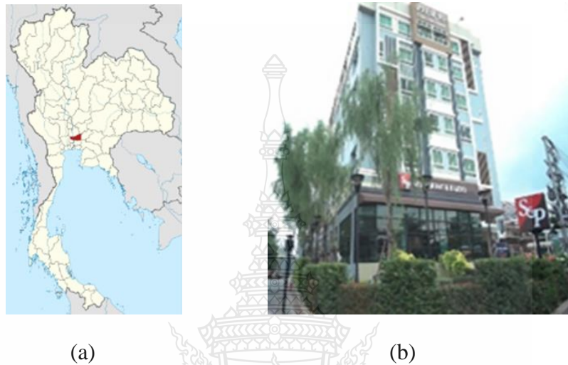
Figure 3.3 (a) Pathum Thani province, Thailand and (b) High-rise PIER 93 building located in the Pathum Thani province
