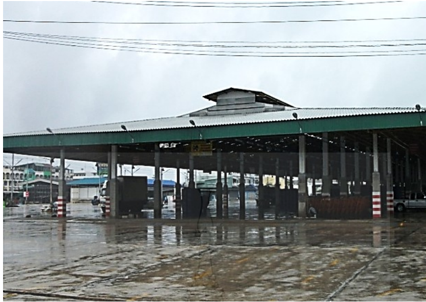
Figure 3.2 The location of PV rooftop system installations used in this thesis.
