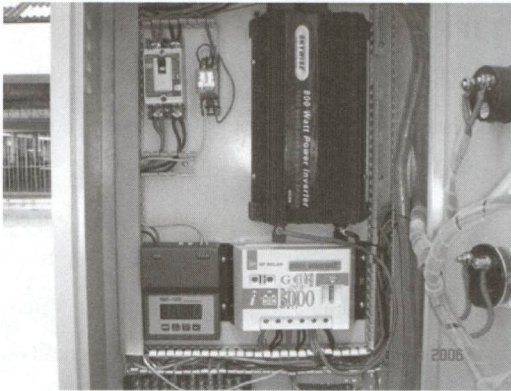
Figure 2 : The control box consists mainly of a controller, an inverter, measurement devices.
