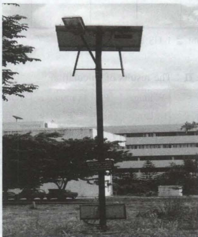
Figure 5 : Solar street lighting system with a high pressure sodium lamp
