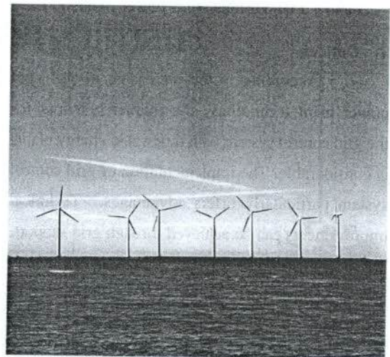
Figure 10 (b): Offshore power plant
