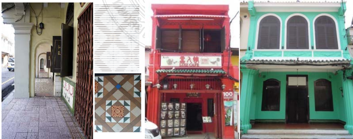
Fig.2 Veranda way & design of floor Fig.3 Rebuild or repainted outside wall of shop-houses
